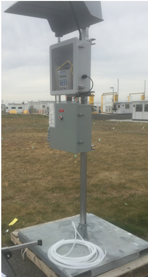
Weatherproof enclosure with solar panel and sun shield
